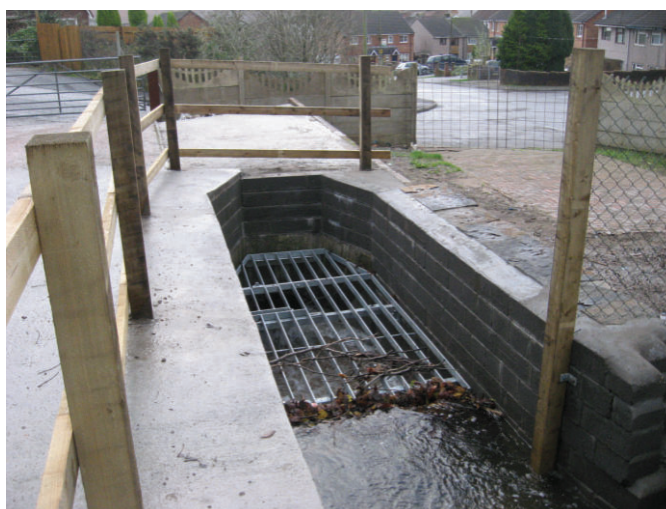
New intake structure
