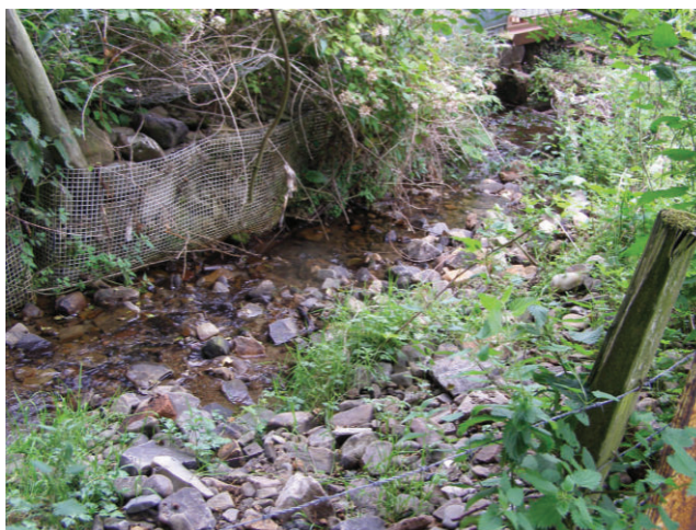
Old intake structure
